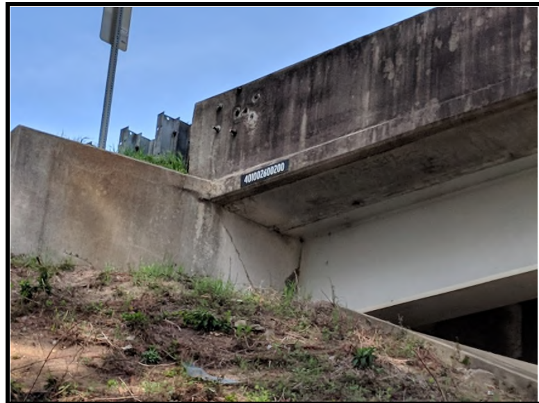
2 The bridge is identified as structure # 401002600200.
