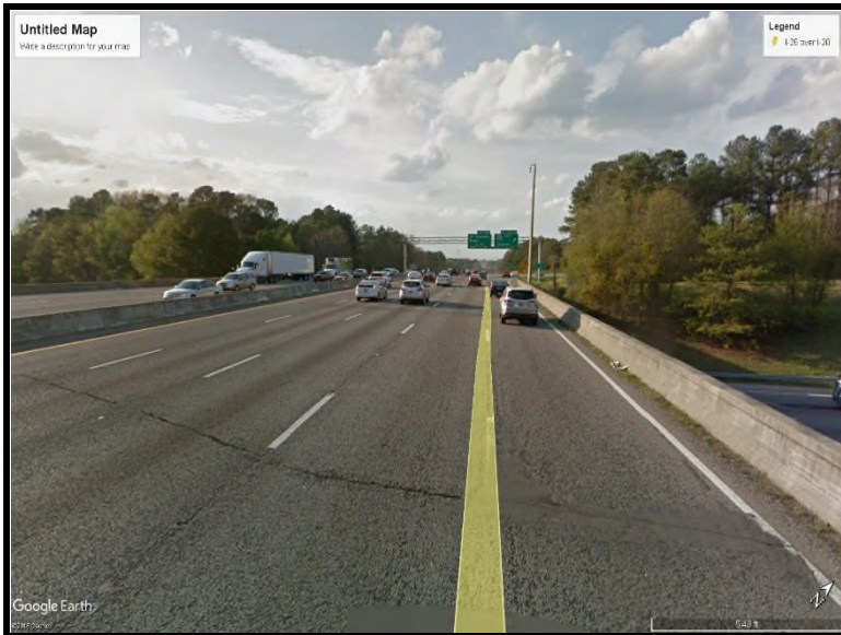
1 View of the I-26 Bridge over I-20 (Source: Google Earth).
