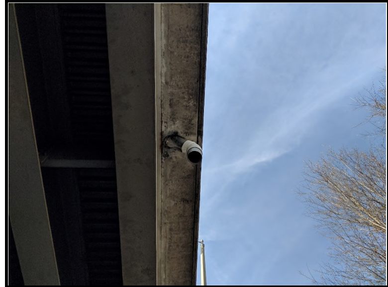
6 Non-suspect scuppers were observed during the assessment of the bridge.
